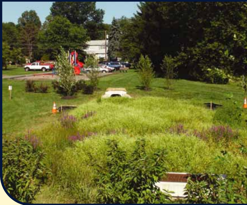
This man-made basin can hold a lot of extra water during a rainstorm
