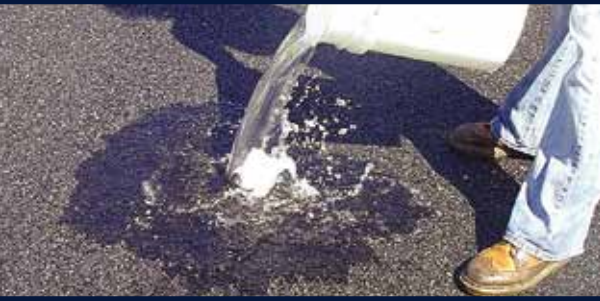
Examples of porous pavement
