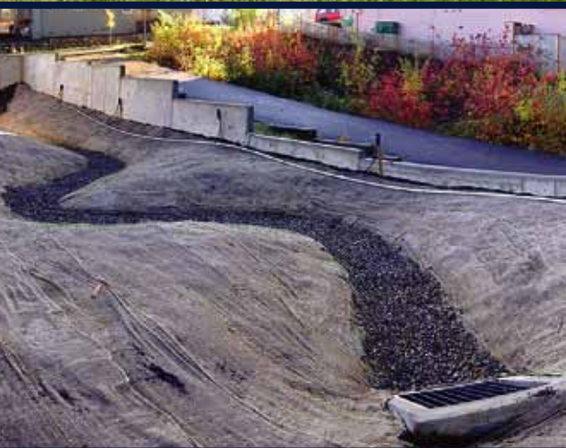
Meandering swale under construction
