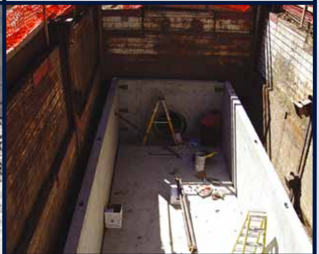
Subsurface system under construction
